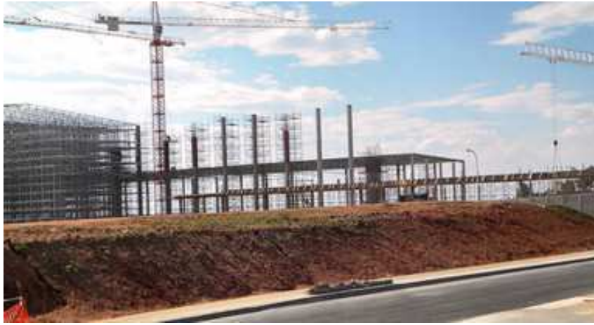
November 2011: 6-storey warehouse under construction
